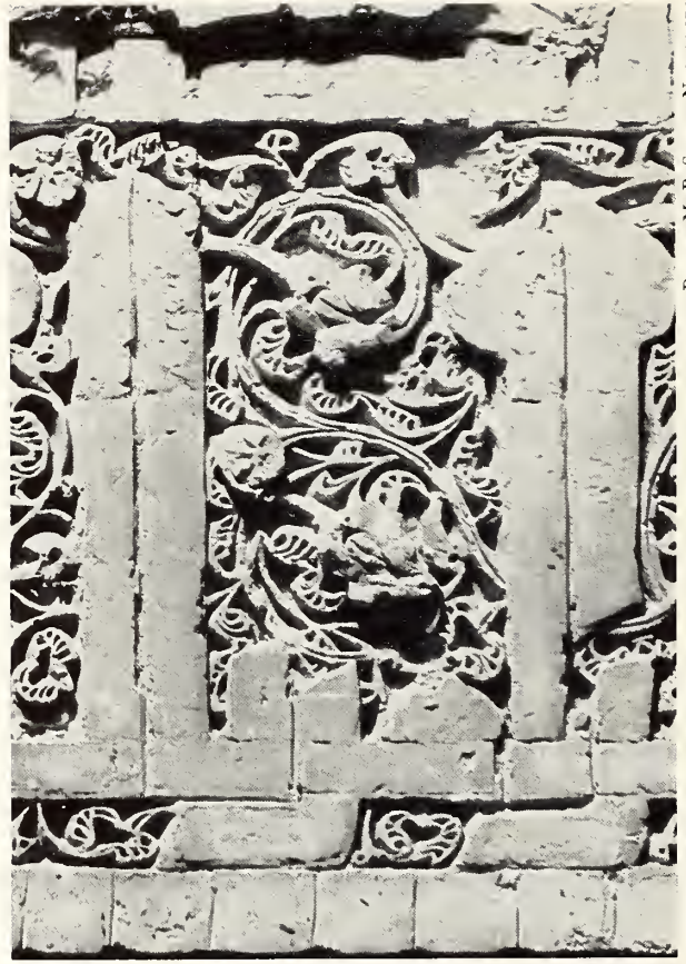
PHOTO, M. B. SMITH, NEG. 770D3 FIG. 31—MIHRĀB, DETAIL OF KŪFĪ INSCRIPTION, BRICK-GAČ REVETMENT
